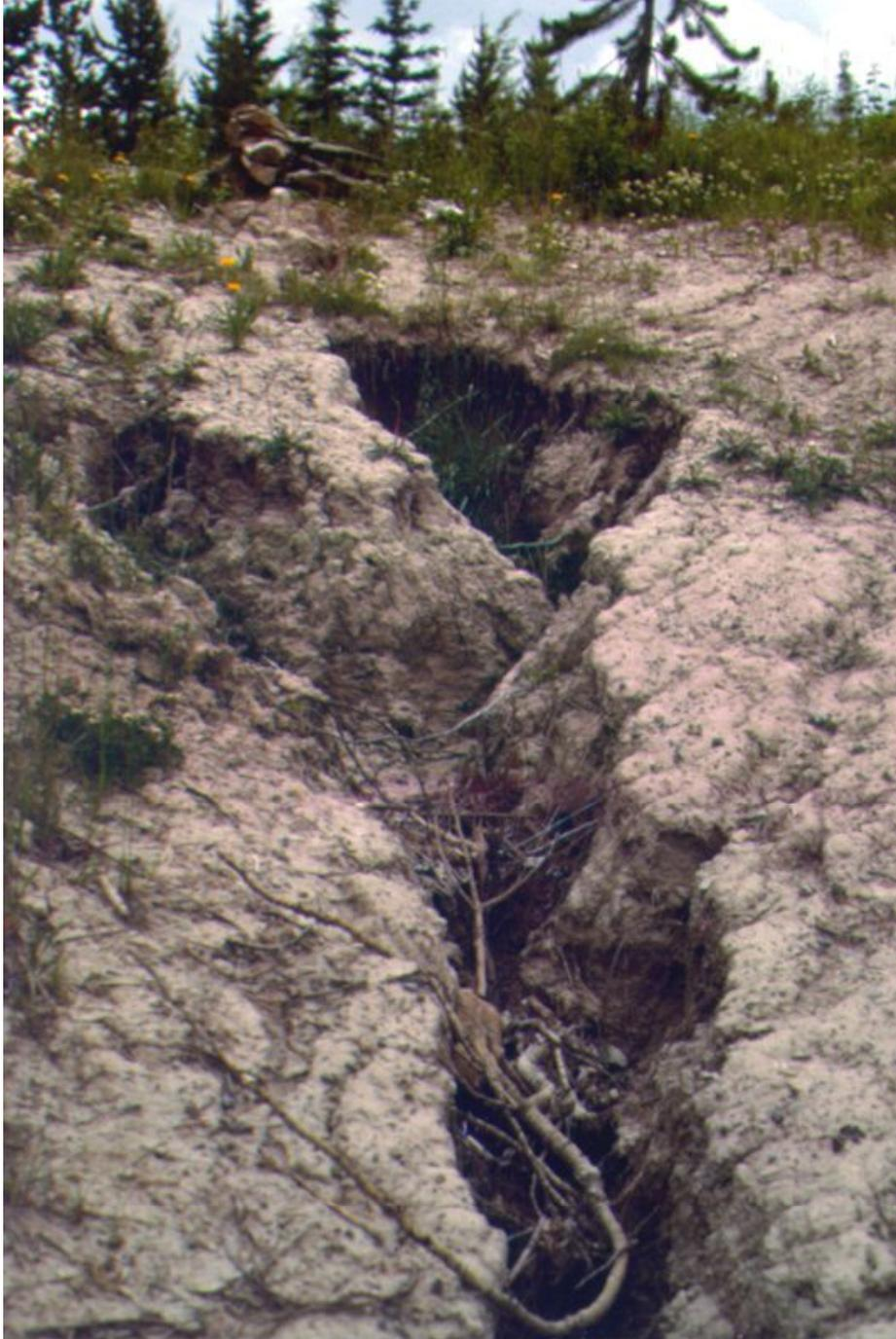
Pipelines take the most direct cross-country routes allowed by the terrain, but are more subject to limitation by topography than are seismic lines. As a result, pipeline problems commonly are due to chronic erosion and mass wasting on the right-of-way (Figure 9), and to direct dumping of fill or dirty ditchwater in streams during construction (Tripp et al. 1992). Instream construction at water crossings is a major source of damage to aquatic habitats from pipelines.
